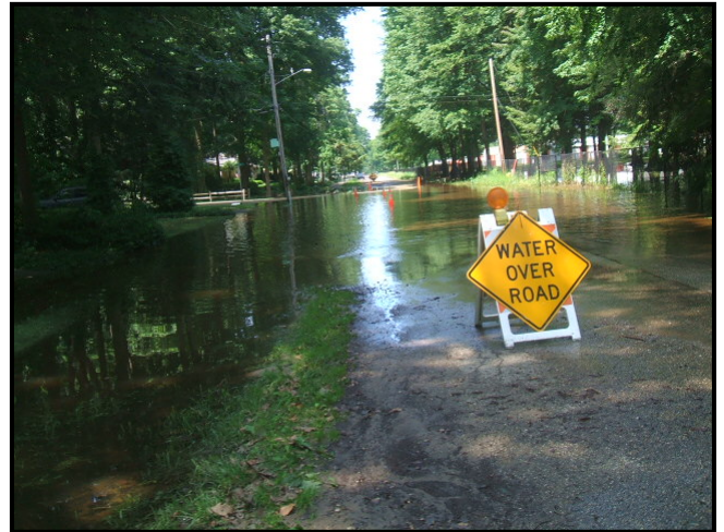
June 2009 Storm Damage
