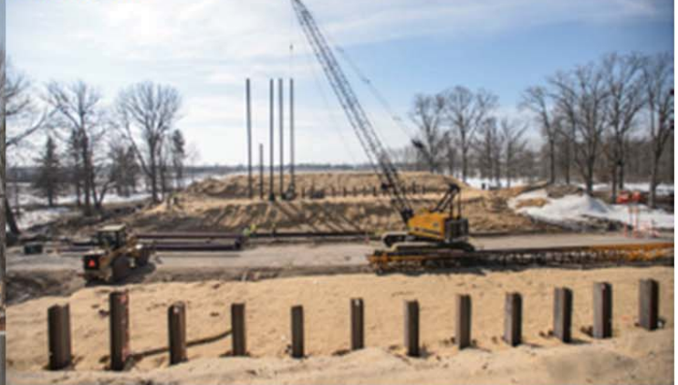
Grand River Bridge March 18, 2014
