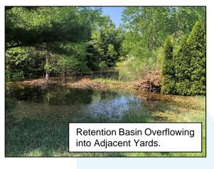
basin. As a result of the high groundwater levels, the retention basin provides virtually no stormwater storage volume below the design high water mark.
