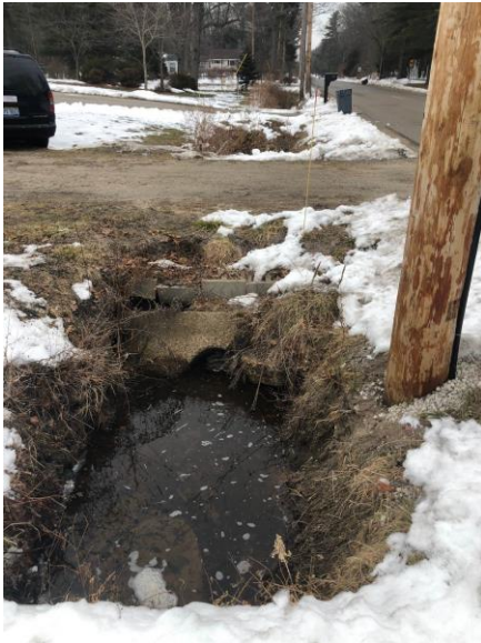
Failing Headwall
