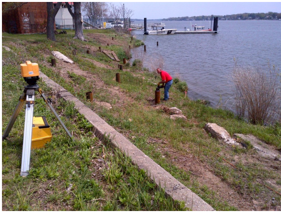
Installing metal pipe piling at new boardwalk location
