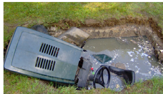
collapsed septic tank lid
