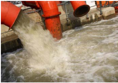
Human (Sewage, Septic tank leakage)
