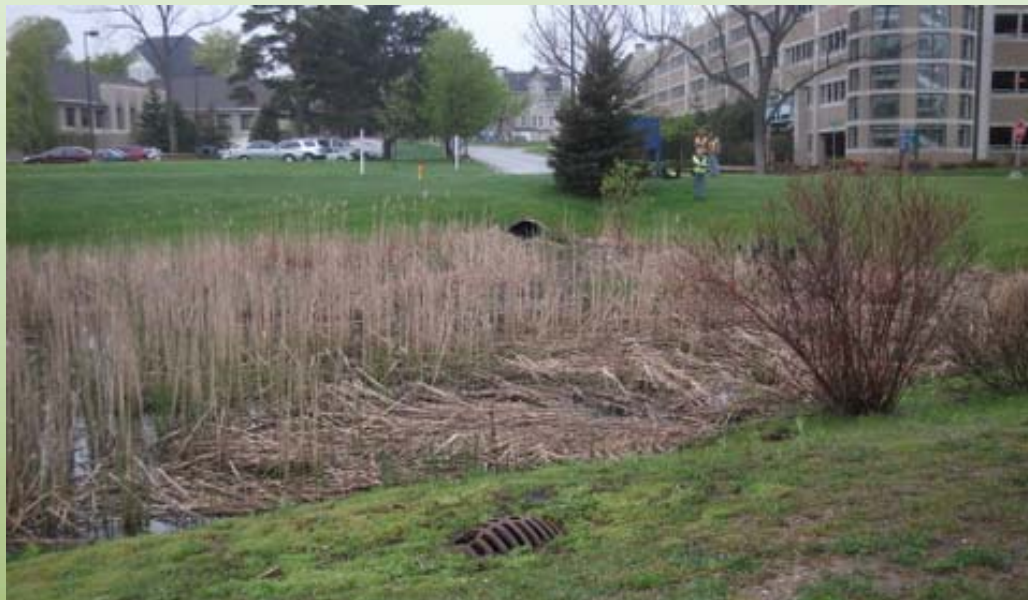
MMC 23 CB at detention inlet to storm drains to 079003
