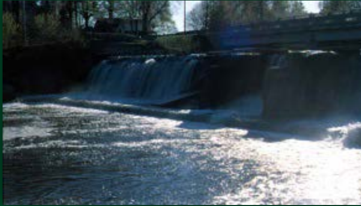
Hubbardston Dam on Fish Creek
