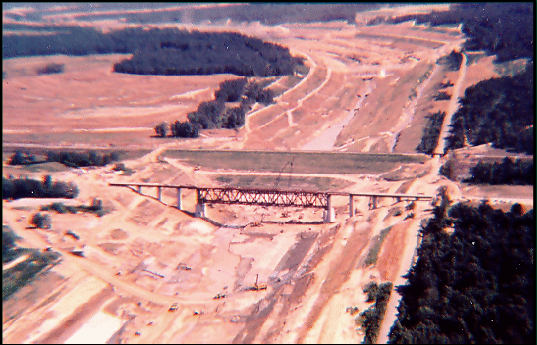
Construction of the Tenn-Tom Waterway (USACE photo)
