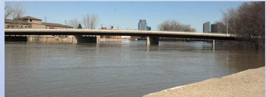
Wealthy St. Bridge
