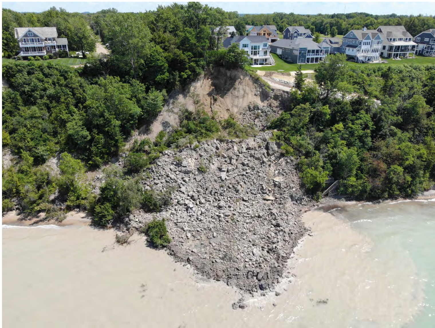
August 29, 2019 failure, Pacific Road and Lakeshore, Miami Park, Picture Sept. 1, 2019
