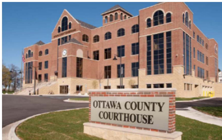
Facilities and Maintenance is responsible for eleven County facilities. The Grand Haven Courthouse, pictured above, is the newest facility which opened in 2009.
