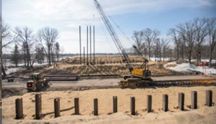
Grand River Bridge March 18, 2014
