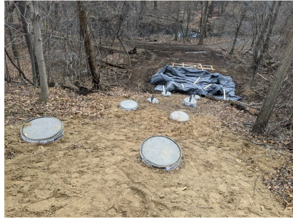
Concrete foundations in place for boardwalk
