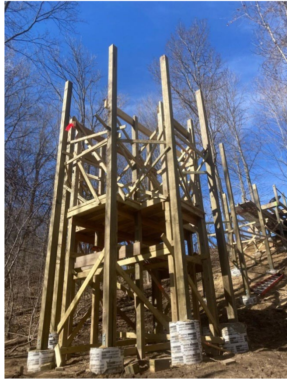
Treehouse support posts in place. Note interior structure is scaffolding. Bottom of treehouse is near the top of the posts
