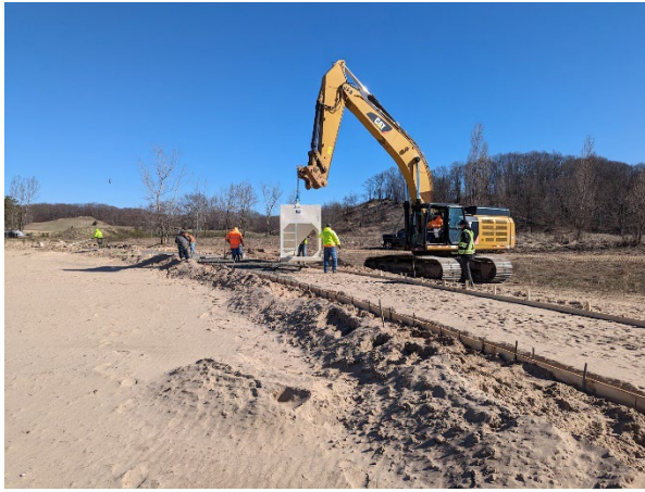
Concrete placement using large equipment
