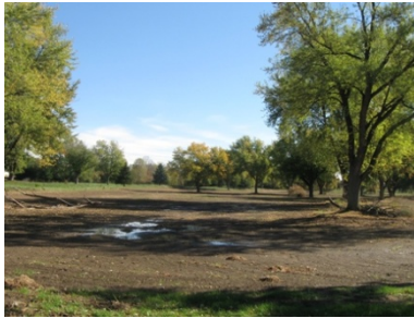
Wetland excavation area
