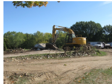
Small building demolished
