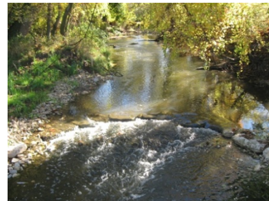
View of rock vane in river
