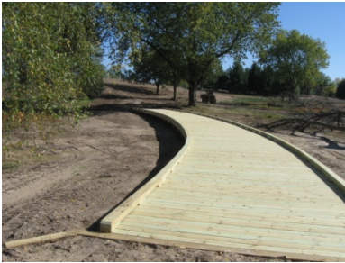
New wetland boardwalk
