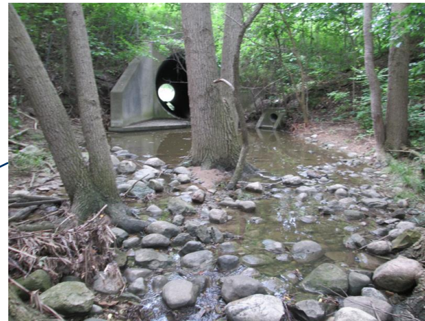
Looking upstream at trees growing in the drain channel just north of the I-196 culvert outlet
