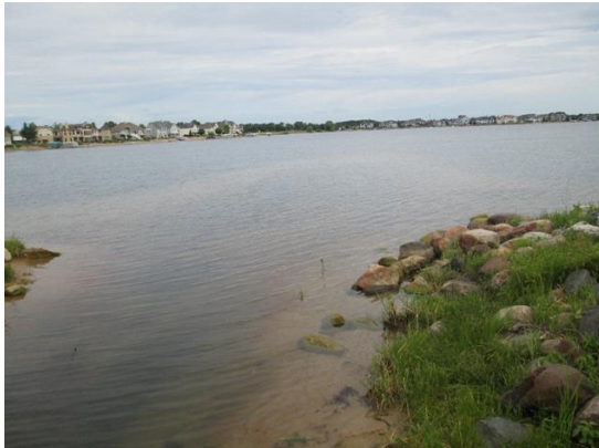
Sedimentation in Georgetown Lake at the outlet of the Corey Bishop Drain (looking north from drain outlet)
