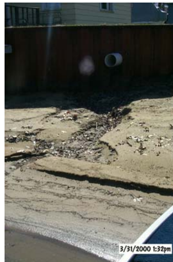
Photo credit: Progressive AE
