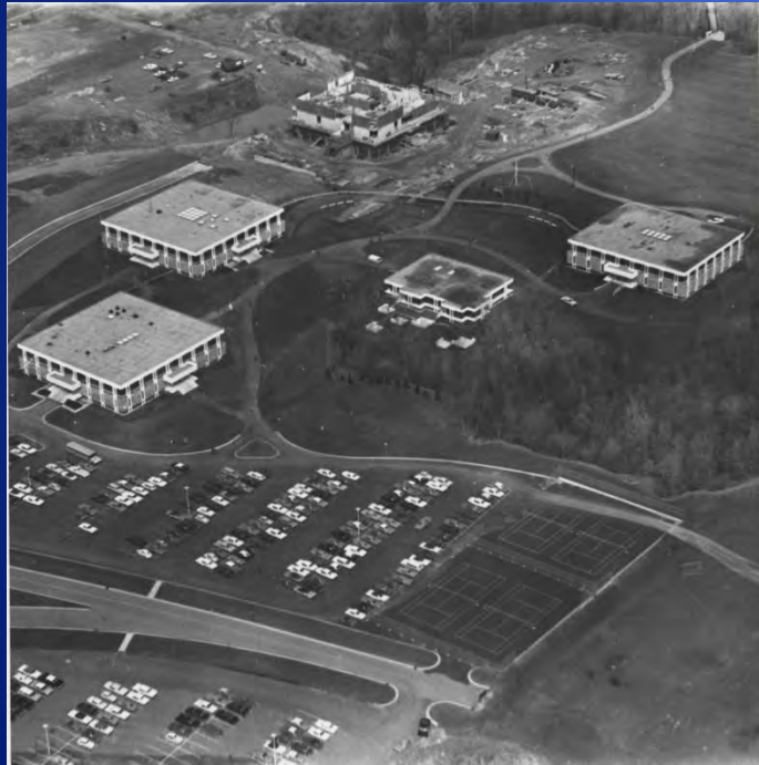
Original library under construction
