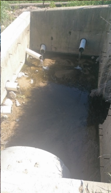
WASCOB Water and Sediment Control Basin
